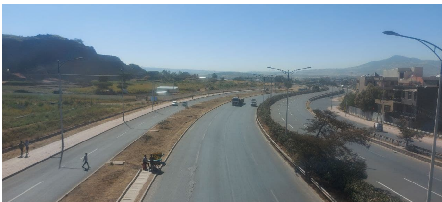
(b) Absence of guiding signs at curves.
