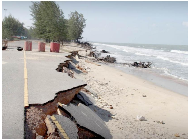
Figure 1.2. The damage of waves on the shoreline in Thailand
