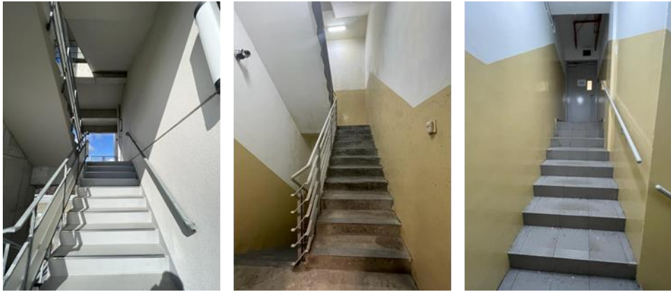
Figure 21. Staircase flights used in experiments – Osaka University (Left), HFT1 L13 (Center), HFT1 B1 (Right)
