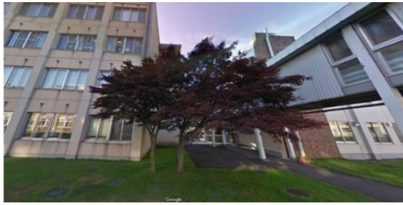
(a) Original image: significant distortion, non-standard viewing angle, and distance.
