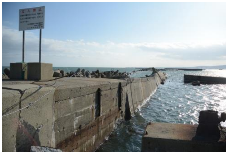
Figure 1.5. Damage to the east breakwater in Iida Port. Caisson collapsed and was submerged in the water. (Sato T., 2024).
